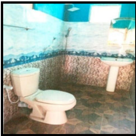
Construction of the toilet system of the Sri Siddhartha Dhamma School in Wariyapola – Awulegama
