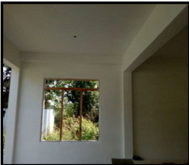
Completion of a part of the Dharmashala building of the Demaladora Sri Nandarama Vihara in the Panduwasnuwara East Divisional Secretariat Division.
