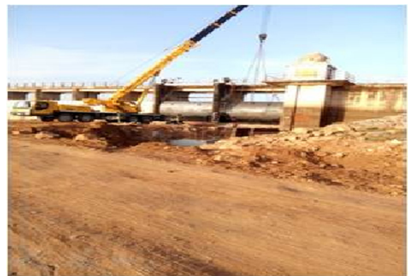
Fixing of a Sluice Gate at Muthiyankaddu Tank
