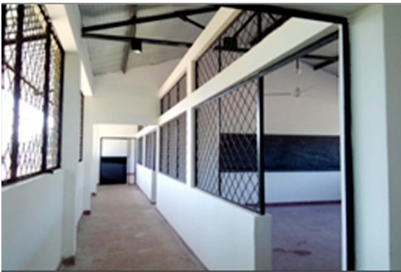
Construction of a School Building - Nagara Maha Vidyalaya
