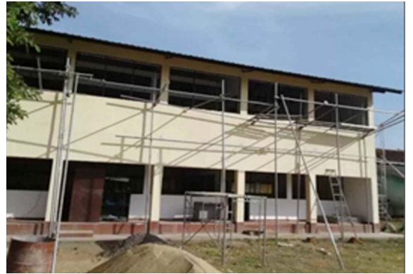
Renovation of School Building at Kaduruwela Nagara Maha Vidyalaya
