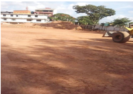
Development Works at Nagananda Temple at Kelaniya
