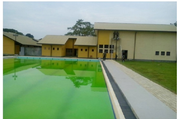
Construction Works at Royal College - Polonnaruwa
