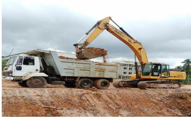
Renovation of Gomarankadawala Mahawewa at Trincomalee
