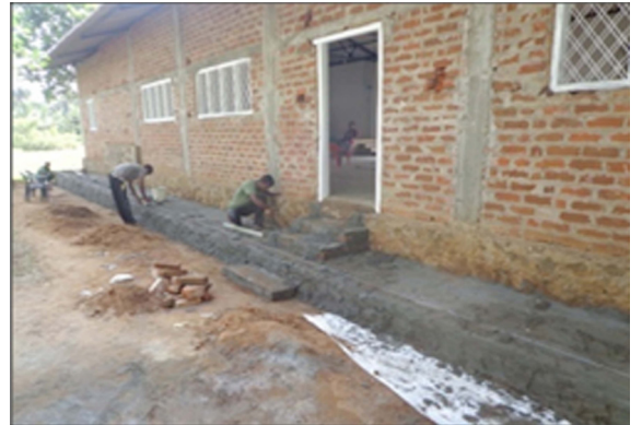
Constructing of a “Preaching Hall” at Unagalawehera Raja Maha Viharaya
