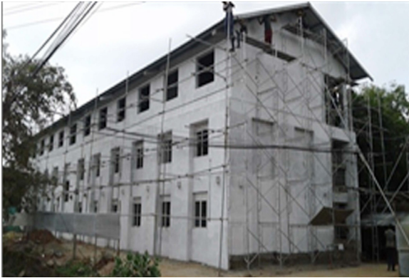
Construction of a School Building - Kaduruwela Maha Vidyalaya
