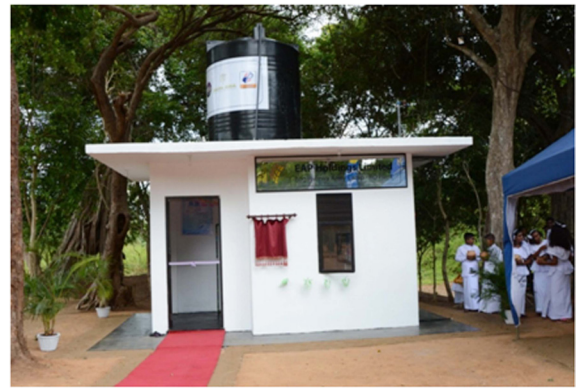
RO Plant - Bogaswewa.
