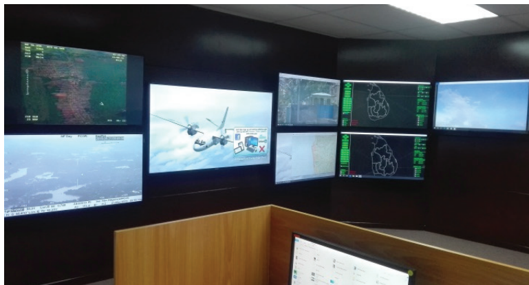
Upgrading of existing Audio Visual System at Battle Management Command Centre
