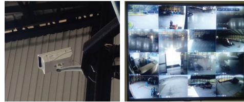
Installation of the CCTV Camera System at No 4 VVIP Squadron Sri Lanka Air Force Base Rathmalana.
