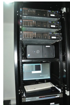
Establishment of the Disaster Recovery Site at Sri Lanka Air Force Base Hingurakgoda.
