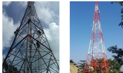
Renovation of the antenna mast at Trade Training School Sri Lanka Air Force Ekala.
