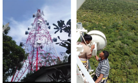
Installation of the PCM link between Madukanda and Recruit Training School Sri Lanka Air Force Vanni.
