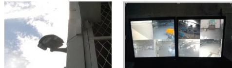
Installation of the CCTV Camera System at No 08 Squadron Sri Lanka Air Force Base Rathmalana.
