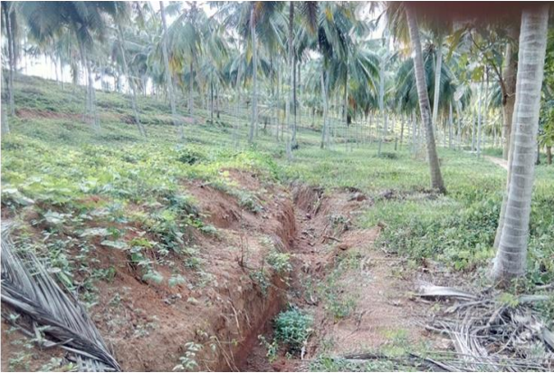
New Draining & Desalting
