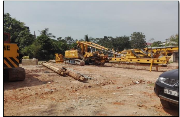
Piling work at the construction site
