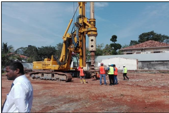
Piling work at the construction site
