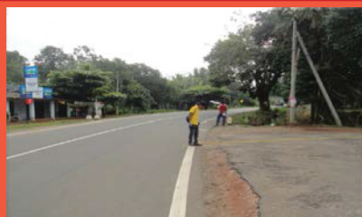
Construction of Mahilankulam Pallaimadu Road
