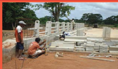
Bridge work Mahilankulam Pallaimadu Road
