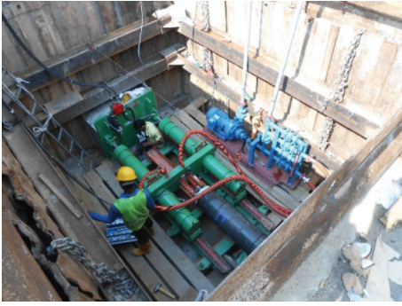
Laying sewer pipes using Micro tunneling
