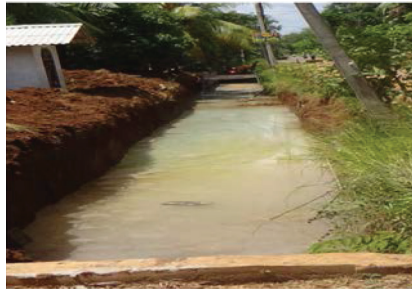
Construction of drainage system, Nagasena Mawatha, Anuradhapura- Rs. 39.95 Mn.
