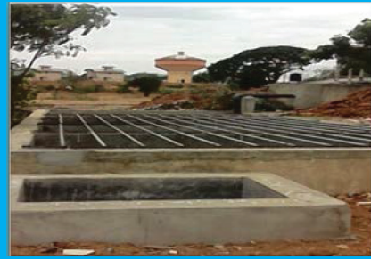
Modernization of gully refine system at Hambantota municipal
