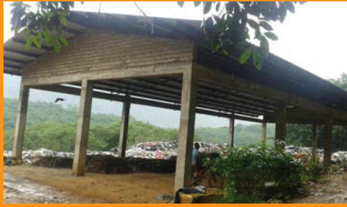
Construction of compost yard in Pradeshiya sabha
