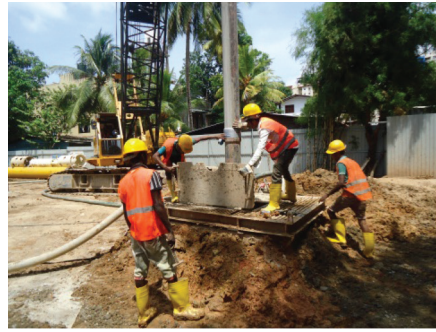
Excavation of Wanathamulla pump station
