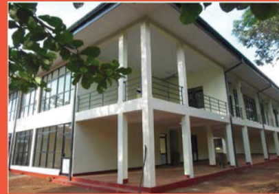
Naula Multi-purpose building
