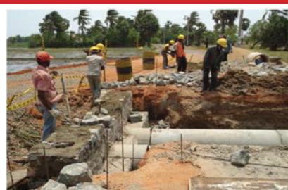
Construction of culverts Uilankulam – Manakulam-Nanaththan Road
