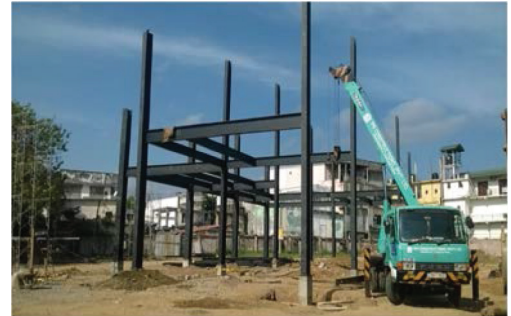
Construction of Ampara Bus stand Rs.280.0 Mn.
