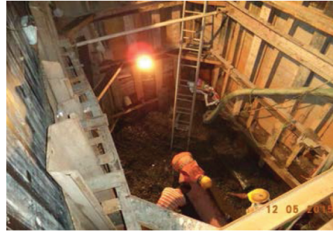
Renovation of Wanathamulla waste water lines
