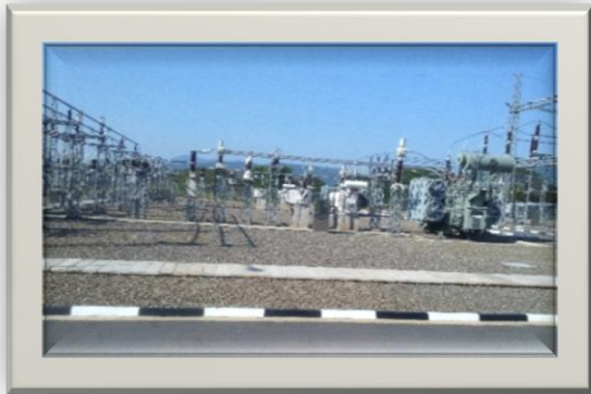
Monaragala Grid Substation
