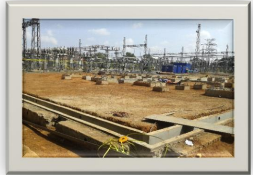
Kilinochchi Grid Substation Constructions
