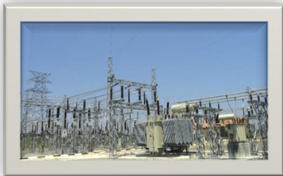
Valachchenai Grid Substation
