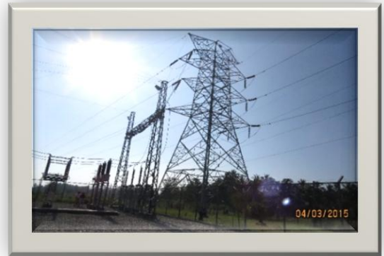
Mahiyangana to Vavunathiev via Ampara Transmission Line
