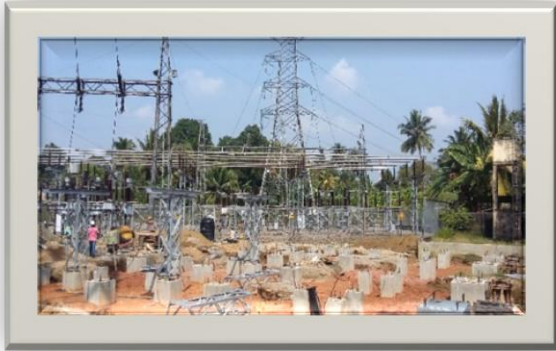
Kelaniya Grid Substation
