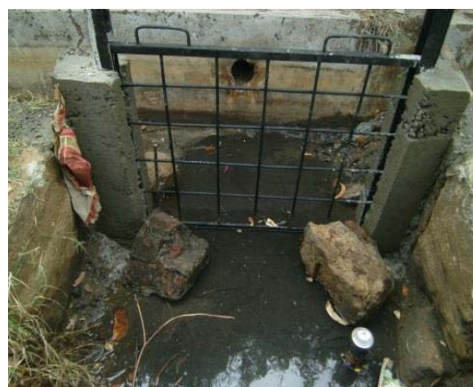
Placing nets to cover the openings of main drainages
