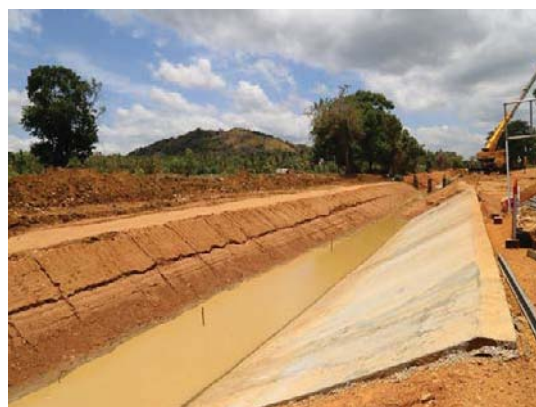
Construction of Main Canal from Wemedilla
