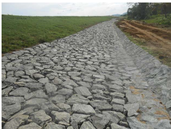
Toe filter and Toe drain in Wan Ela
