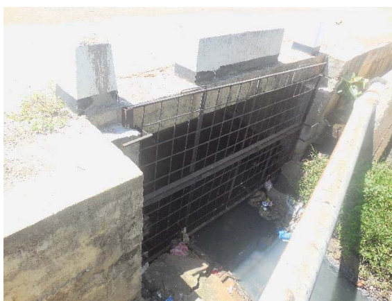
Placing nets to cover the openings of main drainages
