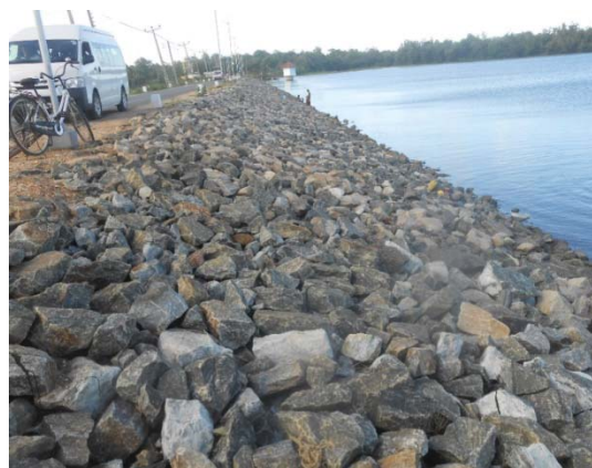
Rehabilitated Rip rap in Bambarawana Reservoir
