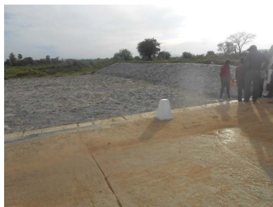
Spillway Down stream protection – Janaranjana wewa
