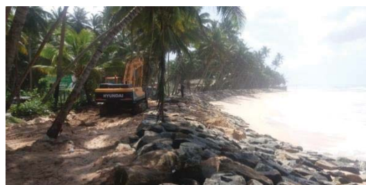
Revetment at Hadiwatta, Habaraduwa after completion.
