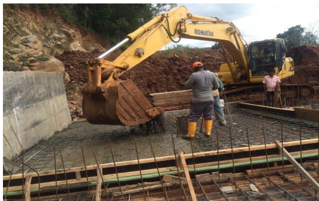
Construction of Spillway
