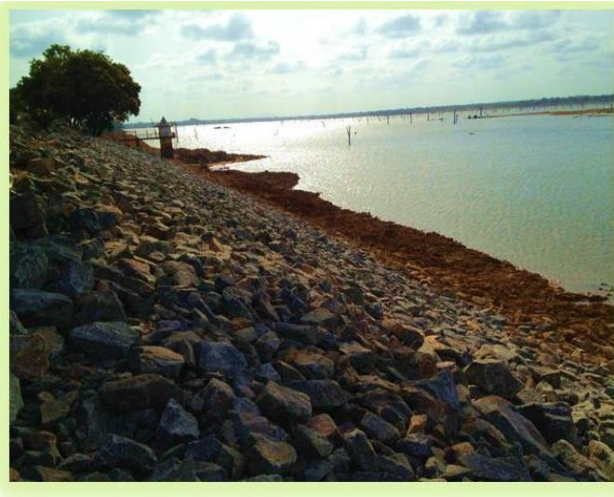
Mahakandarawa Dam – Bund
