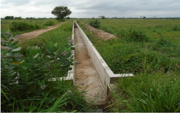
Newly constructed rectangular canal in Radavi Bandi Ela scheme Inginimitiya, Puttalam
