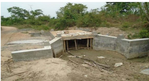
Improvements to G canals in Gonagolla unit in Ampara
