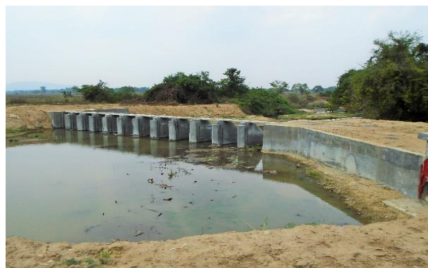
Construction of Shanmugarajah Anicut in Baticalloa
