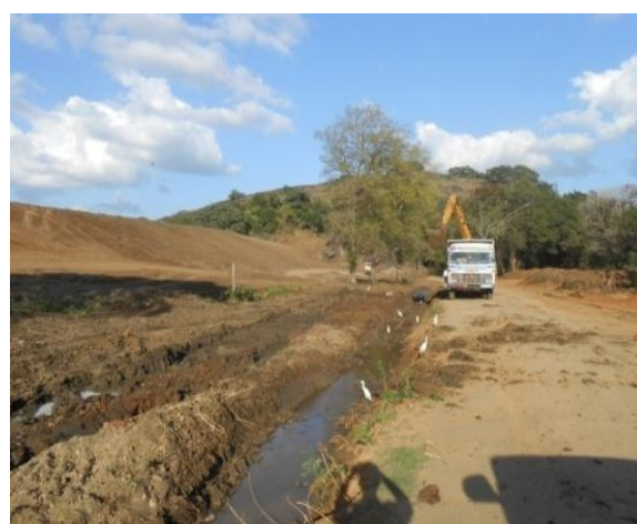
Improvement for Handapanagala Dam
