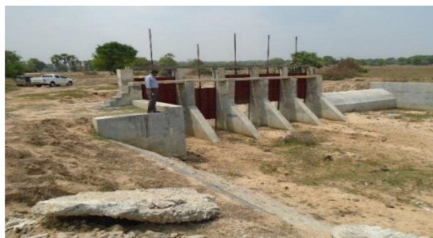
Construction of Kayanmadu Regulator in Baticalloa
