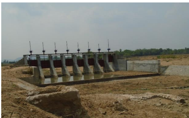
Construction of Nelluchchenai Anicut in Baticalloa
