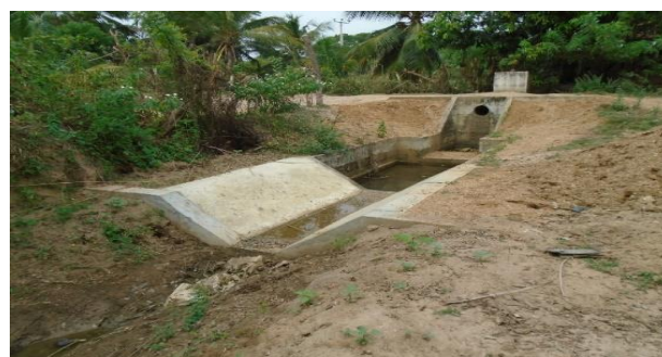
Construction of drop structure G 23.1 Canal in Gonagolla unit in Ampara
