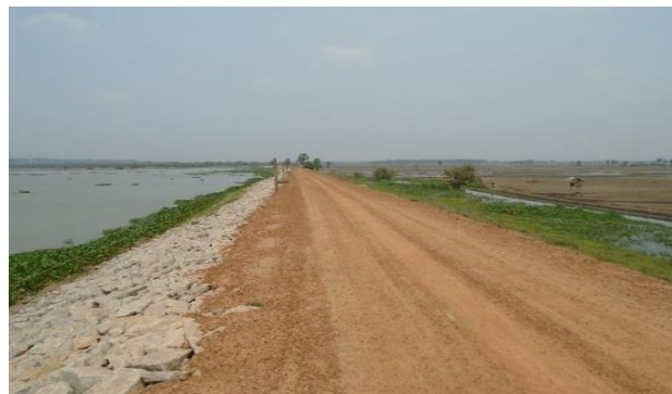
Reconstruction of Anaivilunthan Anicut in Neethai River in Illukuchenai unit
