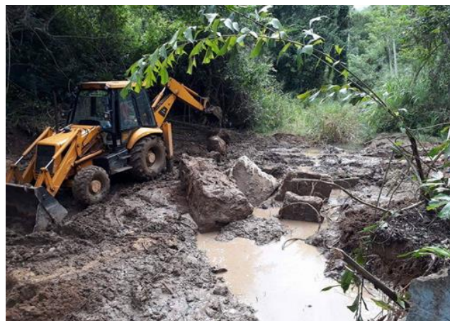
Clearing and construction works of anicut (Magandana Scheme – Monaragala)
