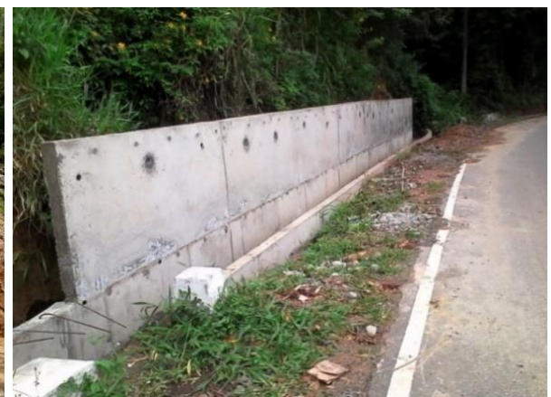
Construction of lined drain with raised concrete wall and gabion wall in Kottagoda podumilla yalagamuwa road
