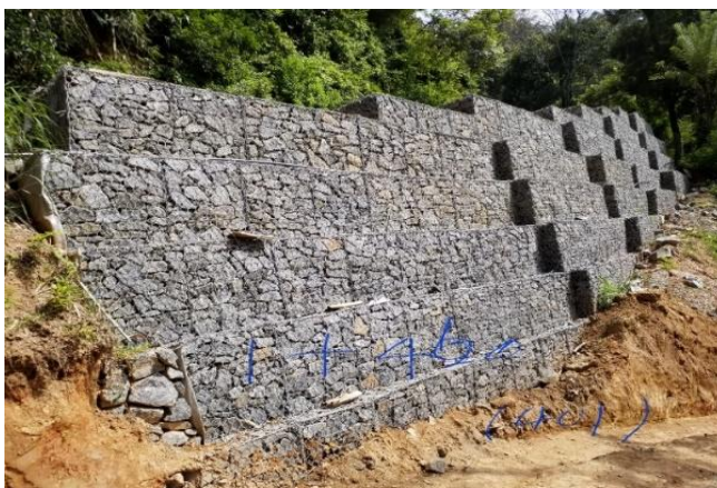
Construction of lined drain with raised concrete wall and gabion wall in Kottagoda podumilla yalagamuwa road
