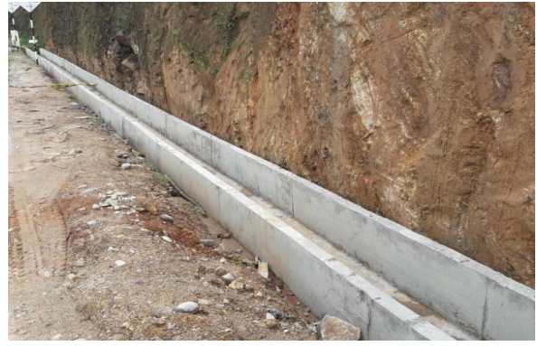
Construction of concrete U drains in Kottagoda Podumilla Yahalagamuwa Road
