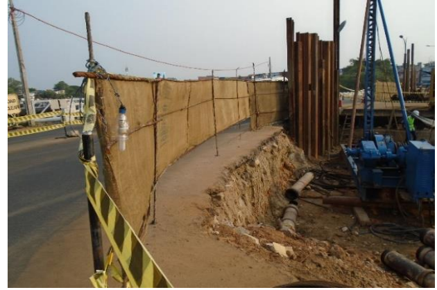
Construction of Koddamunai Bridge (1/1) on Batticaloa - Trikondimadu- Trincomalee Road
