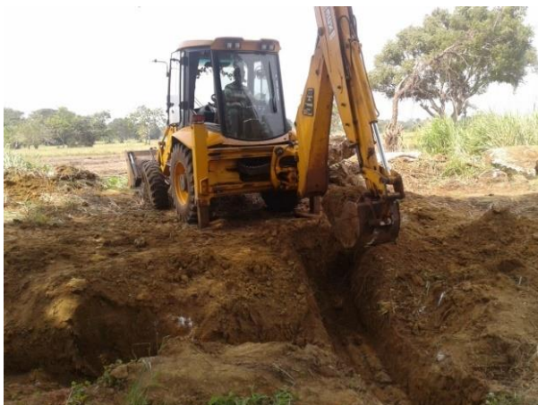
Constructions of field canals (Manankattiya Scheme)
