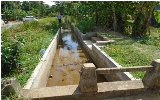
Canal lining with bathing steps in Inginimitiya scheme
