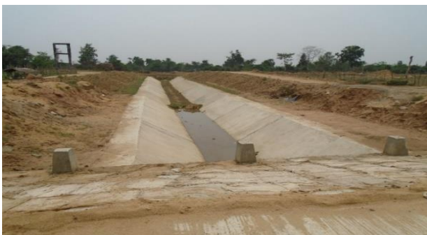
Construction of Palamadu channel Rugam scheme in Baticalloa
