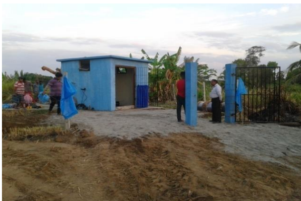
Figure 18: Construction of Pump House at Pallegama
