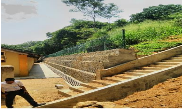
Retaining wall behind a school building at Galkanda Kanista Vidyalaya
