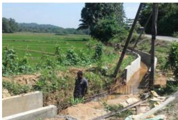
Canal under construction (Diyalape Amuna Scheme - Matara)
