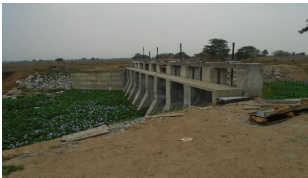
Improvements to Valathapitty tank & Improvements to spill tail canal to prevent flood damage in Moravil I unit
