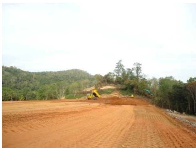
Construction of Alikota Ara Dam
