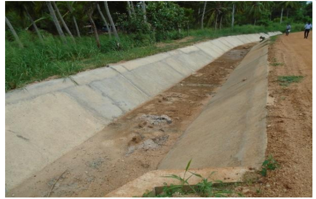
Canal lining Improvements to RB main canal in Inginimitiya Scheme
