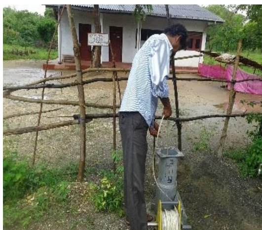
Figure 11: Rehabilitation of a hand pump
