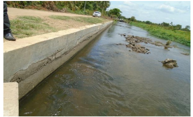
Construction of retaining wall in D1 canal in Ranketha D1 off LLMC & in LLMC
