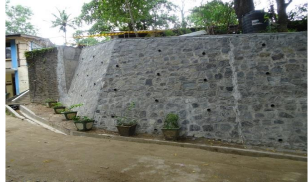
Retaining wall at Sirimalwatta Navodya vidyalaya
