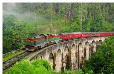
Nine Arches Bridge
