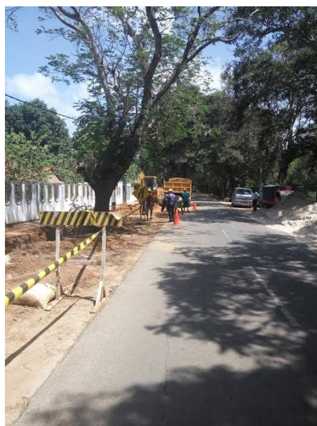
Pump laying for sewerage –02 Zone Sella Road
