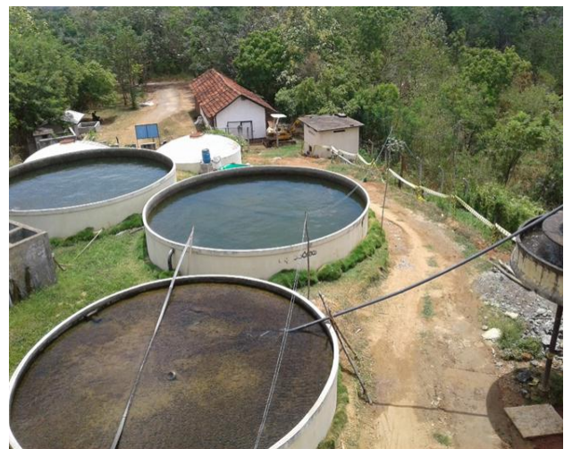
Gangeyaya WSS (Rehabilitation) in Rathnapura District
