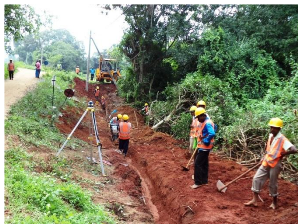
Lot C1 Contract Package - Pipe laying work at Medawachchiya Area
