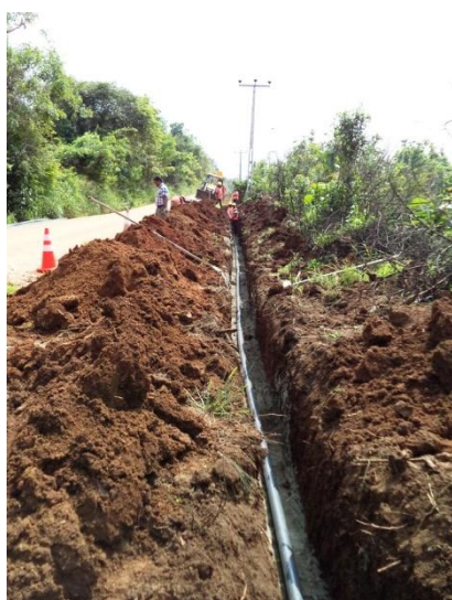
Lot C3 Contract Package – Pipe laying work at Ethakada Area
