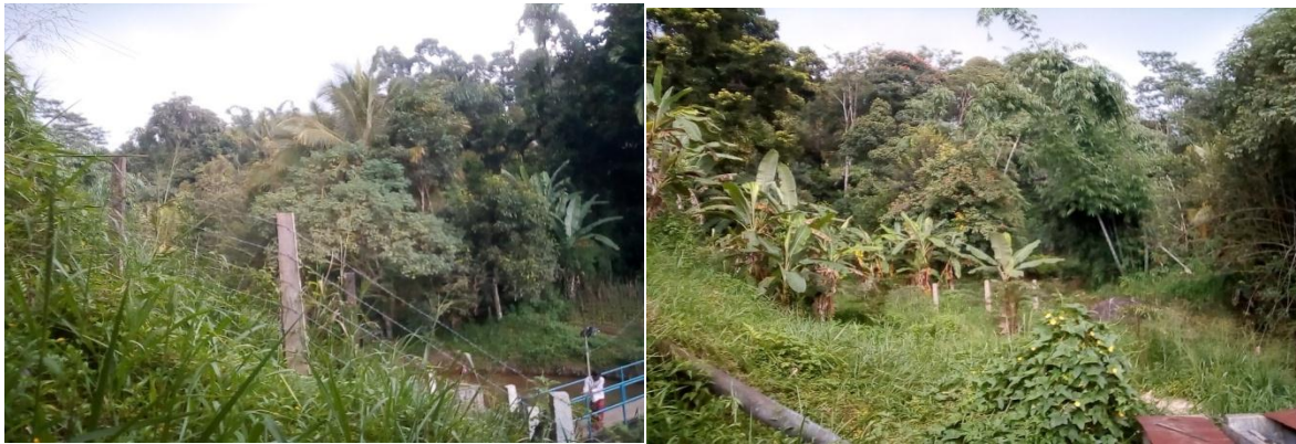
Intake protection fence for Paradeka water supply scheme
