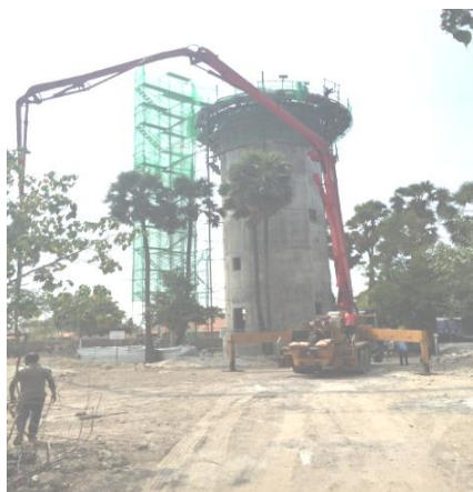
Water Tower at Punguduthivu
