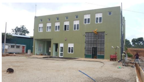
Puttalama Treatment Plant
