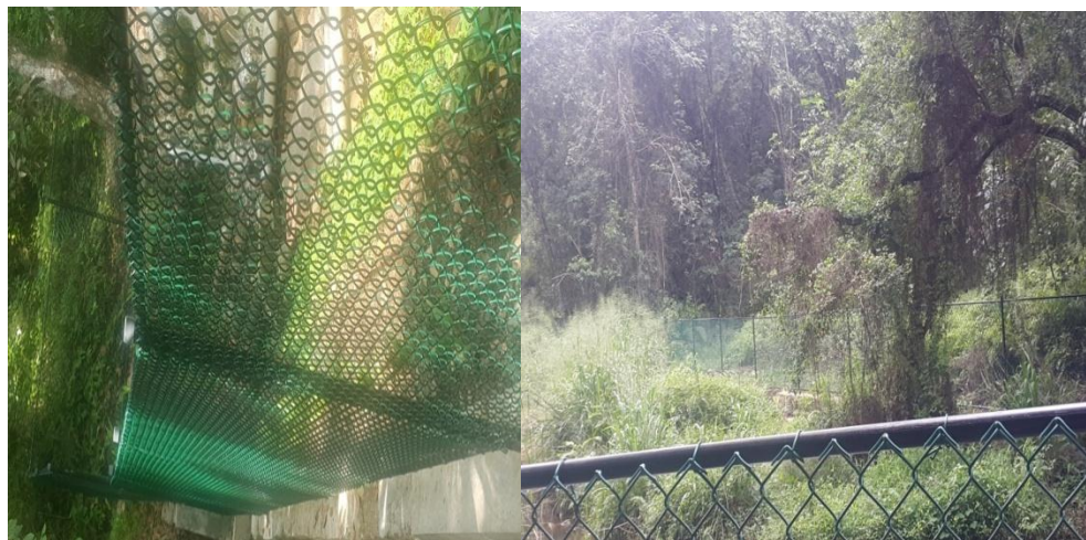
Chain Link Fence around water source- Kahawatta and Nivithigala wss
