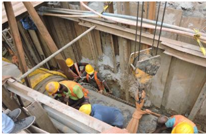
Un-expected underground utilities during the construction
