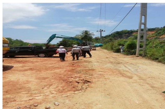
Construction work is started in Salinity Barrier
