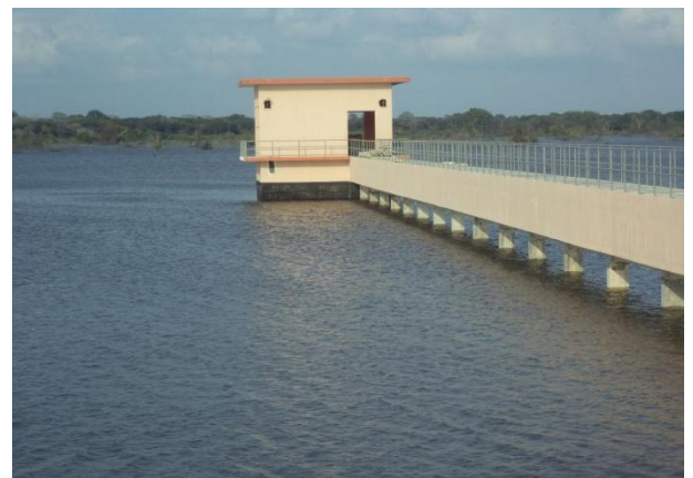
Intake and Water Treatment Plant
