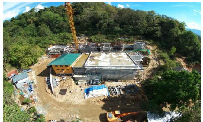
Kumbukkana Water Treatment Plant
