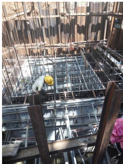
The Pump house is being built
