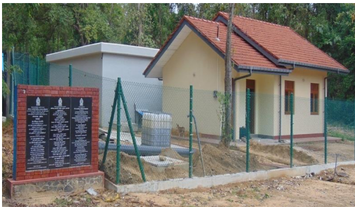
Under Ground Reservoir in Kumbukkana and Operetor's Quarters
