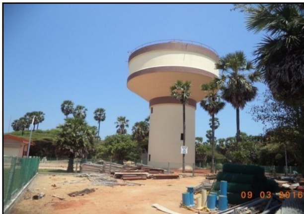
Water Tower - Elthur
