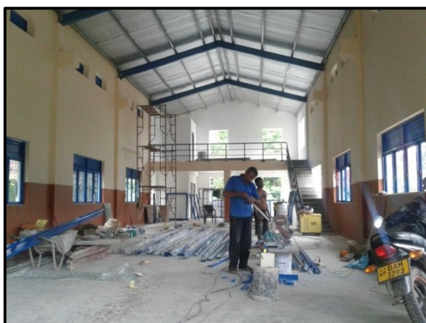
Construction of buildings in progress
