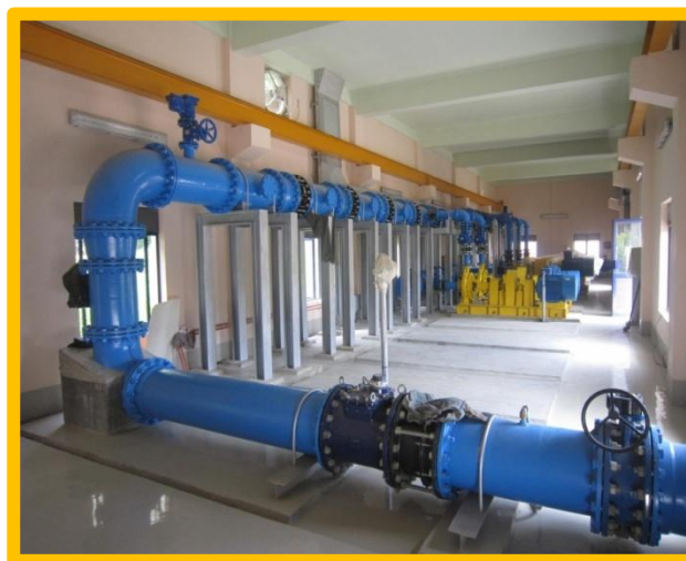
Yatiwawala Pump house
