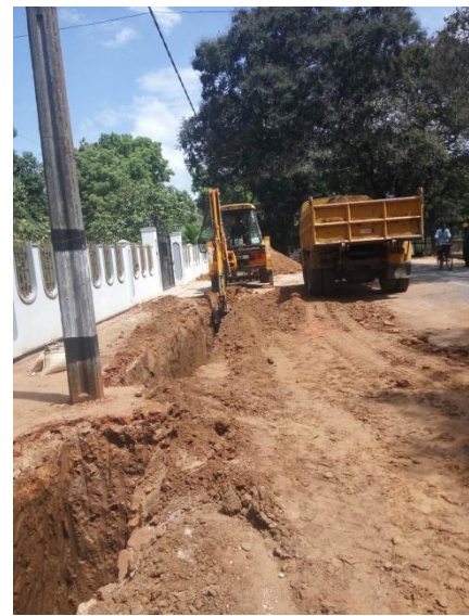
Excavation of drains for laying the pipeline Region -2 – Sella Road
