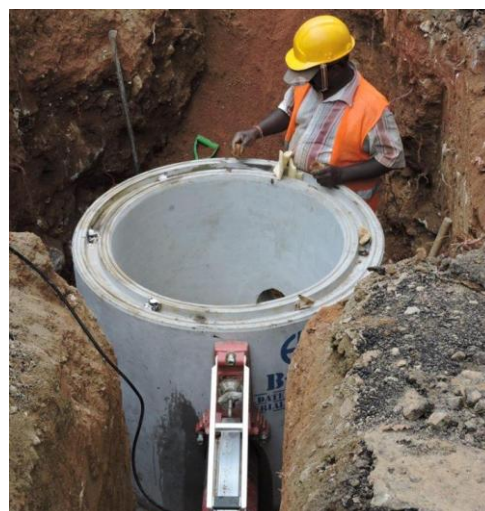
Construction of Manholes in Heeressagala First Lane
