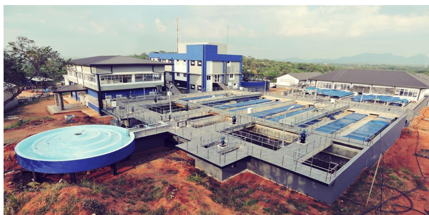
Water Treatment Plant
