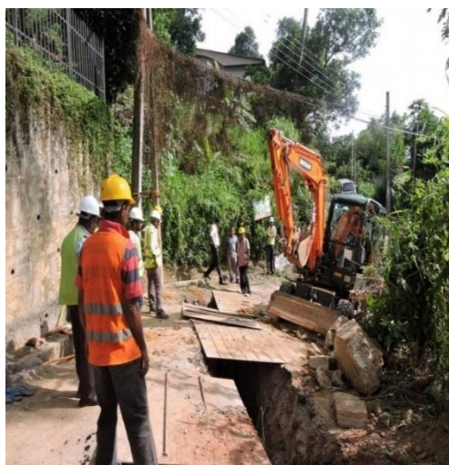
Blasting in progress for laying pipeline in Heeressagala First Lane
