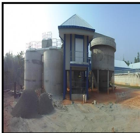
Mud Depositor and Lime Collecting Tank which are being built.
