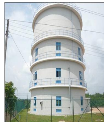
Welmilla Water Tank
