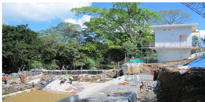
Okkampitiya Intake and Water Treatment Plant
