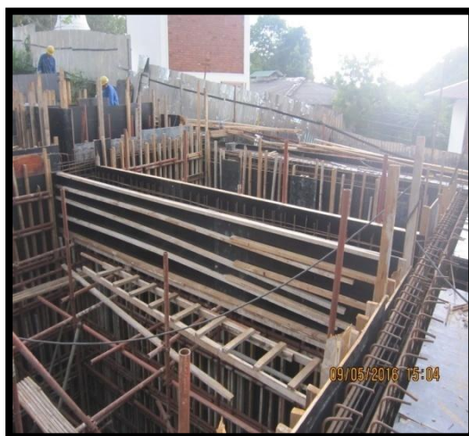
The Water Treatment Plant is being built
