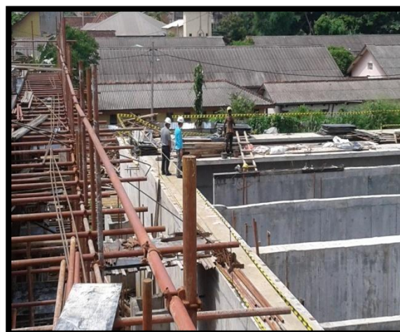
The Integrated Tank is being built
