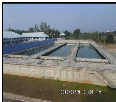
Completed Water Treatment Plant
