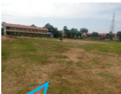
Al Azhar School ground renovation
