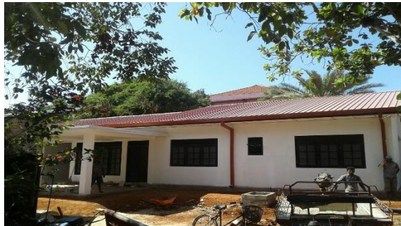
Construction of Quarters for DS Mannar
