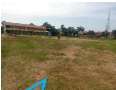
Al Azhar School ground renovation
