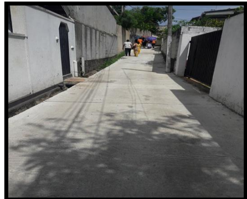
Divisional Secretariat: Dehiwala Project: Laying concrete of the byroad starting from No. 5A to 23/3 in Medhankara road.
