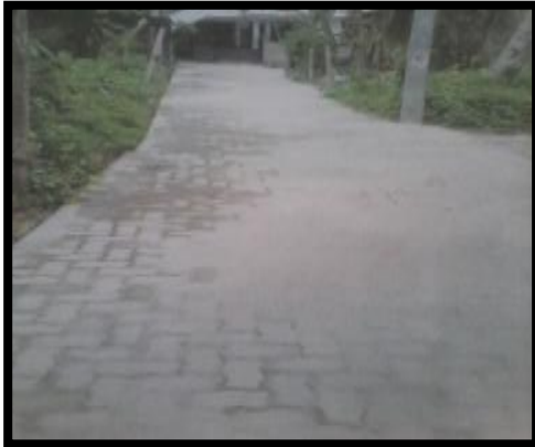
Divisional Secretariat: Maharagama Project: Developing the remaining part of Nisala uyana road in Neelammara road, Katuwawala
