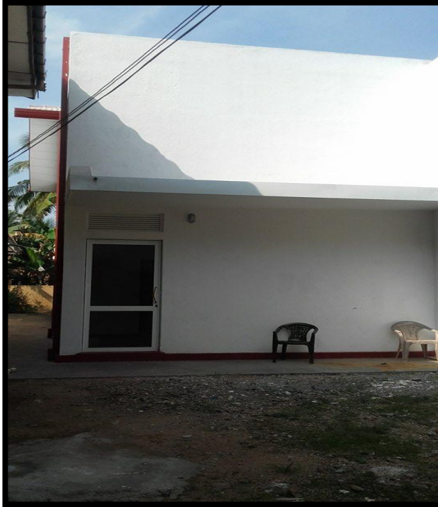
The side view of the building
