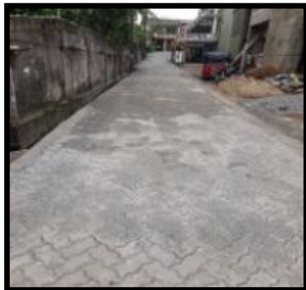
Divisional Secretariat: Kotte Project: Developing and interlocking the byroad from public well at Stanly Thilakarathna mawatha to Pelawaththa road
