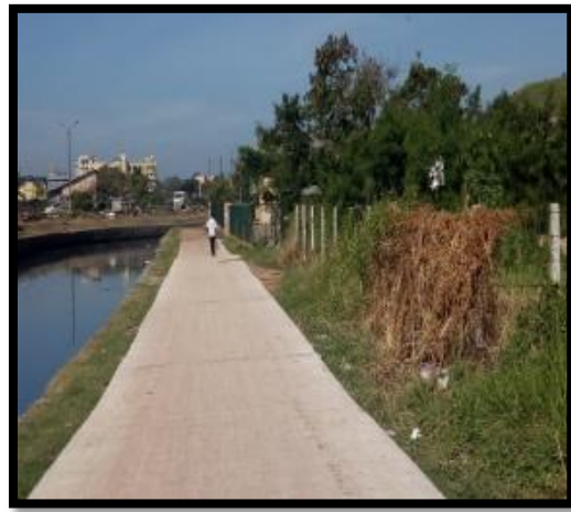
Divisional Secretariat: Colombo Project: Concreting the access road for city Jayamaga Sewana housing scheme in Sirimawo Bandaranayake mawatha, Colombo 14.
