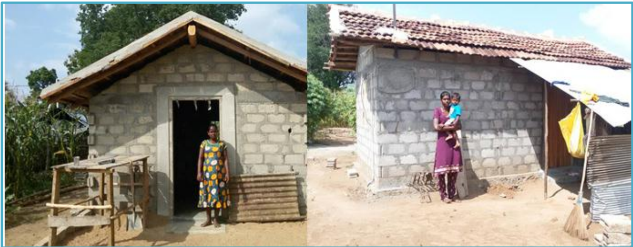
Construction of New Houses- Koralapattu South
