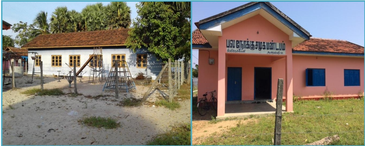
Repair works - Divisional Sewapiyasa Buildings of the District- Eravurpattu & Manmunai Divisions
