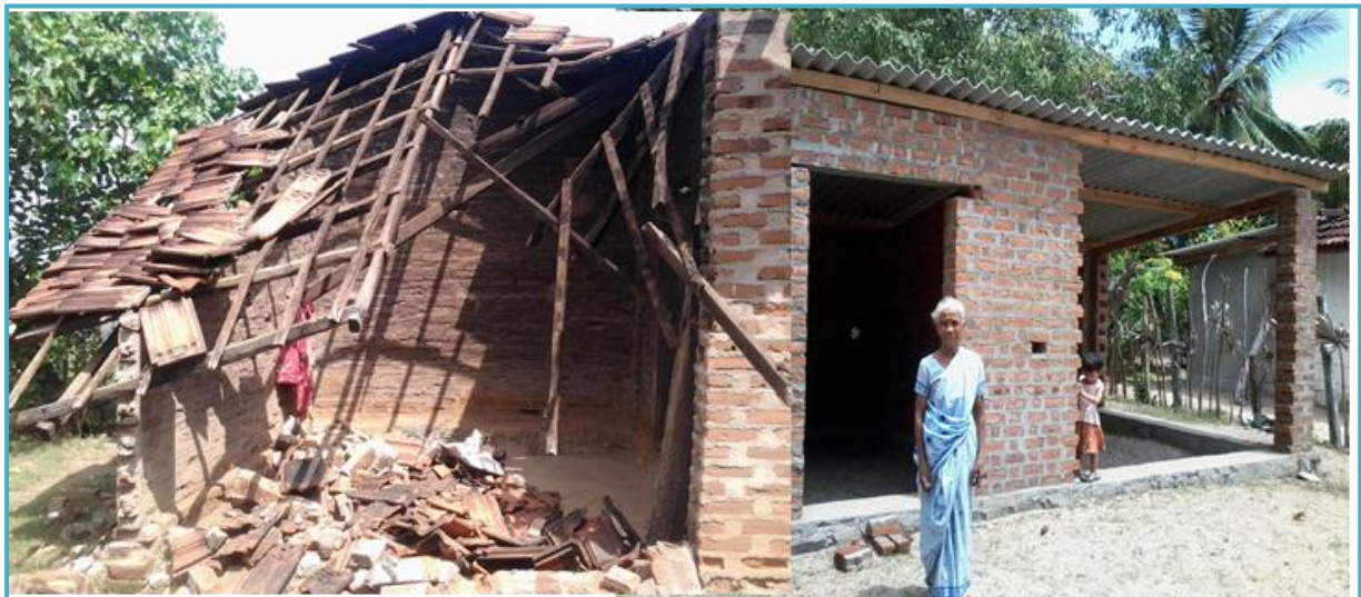
Partly repaired Houses- Manmunai south Eruvilpattu
