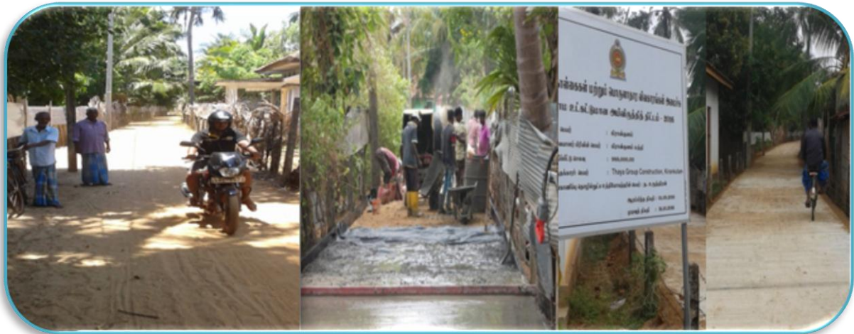
Const. of Concrete Road & Drainage – Sewing Centre Road, Kirankulam, Manmunaipattu
