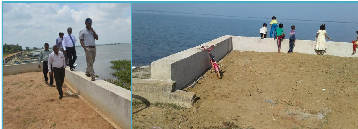
Retaining wall at Kankeyanodai –Manmunaipattu Division
