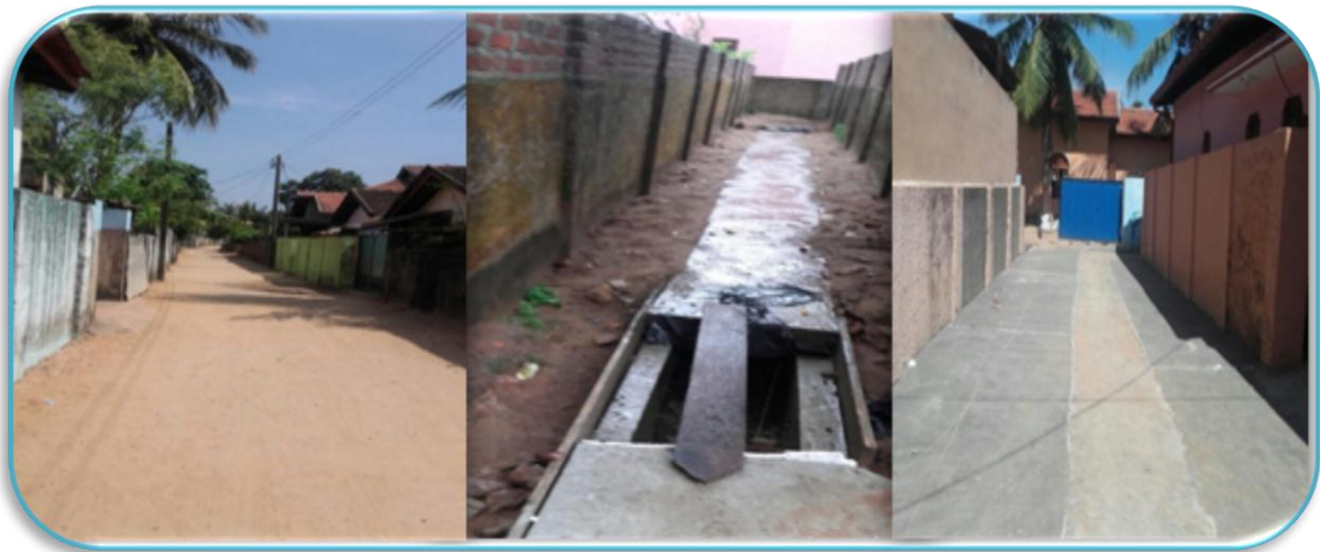
Const. of Concrete Road & Drainage – Hashra St., Koralaipattu West, Oddamavady
