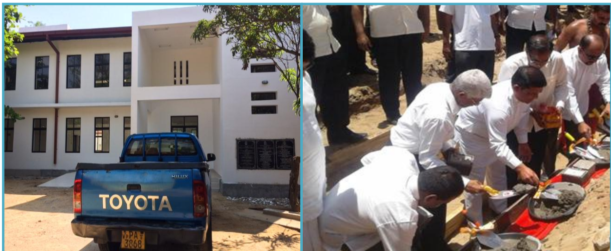
Laying foundation stone for Partly Secretariat building at Manmunaipattu
