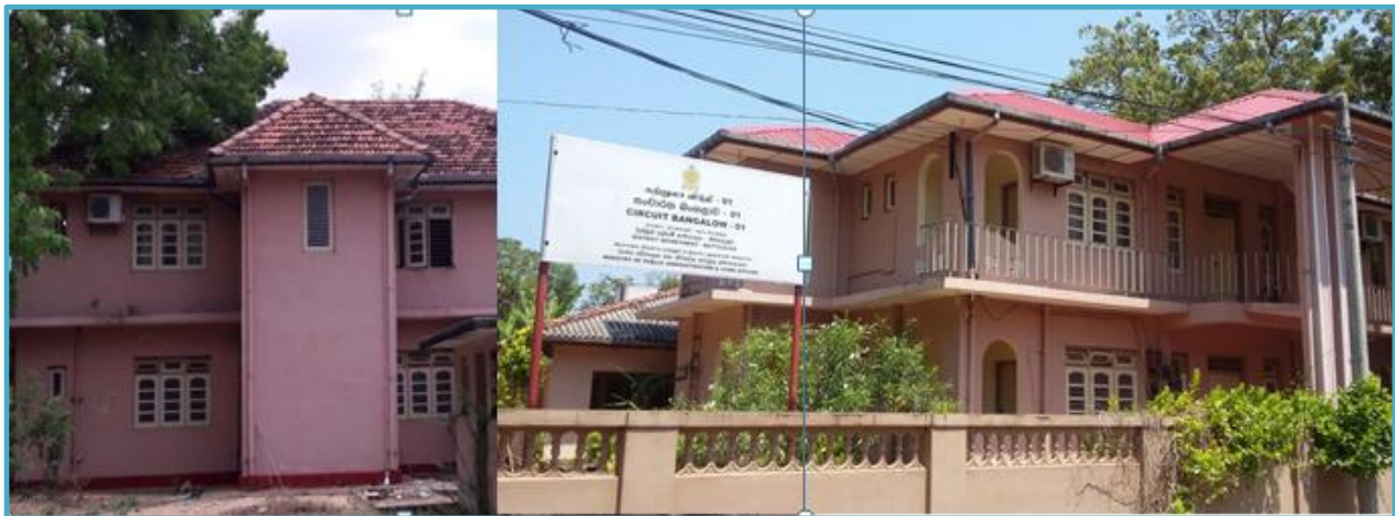
Repair works - No.1 Circuit Banglow Building, Kallady
