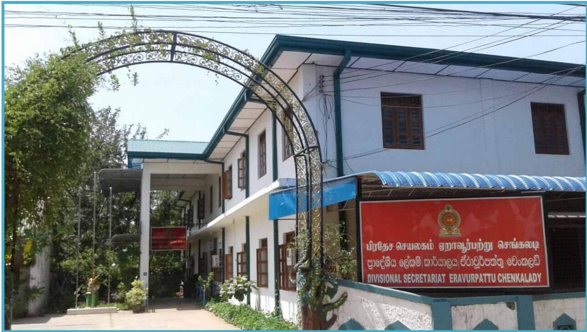
Repair works - Divisional Secretariat Building, Eravurpattu-2016
