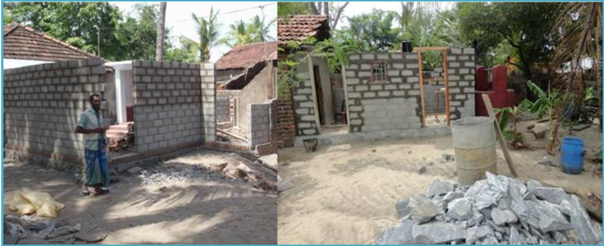
Construction of New Houses- Koralapattu Central
