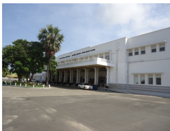
Completed Jaffna railway station
