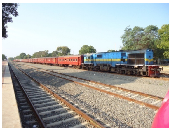
Completed Northern rail track
