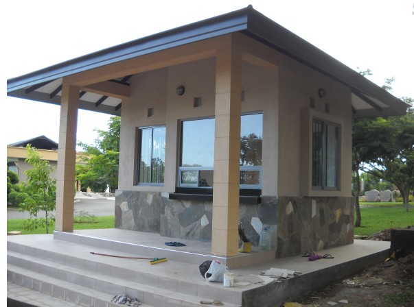
New entrance ticket counter with a fence has been constructed in the front entry part of the garden
