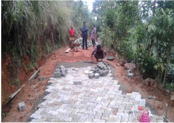
(Matara District Road construction in the model village)
