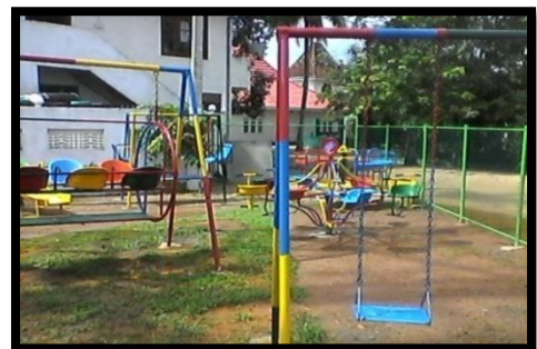
Project: - Building Children's park in "Thisarana" Preschool of Sri Dharmawijayaloka Viharaya
