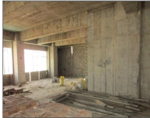
Block works for walls of 11th floor
