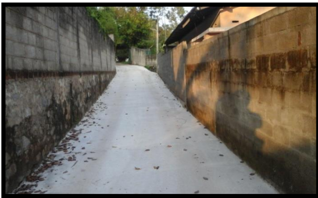
Projects:- Developing Nagaha road – Maharagama
