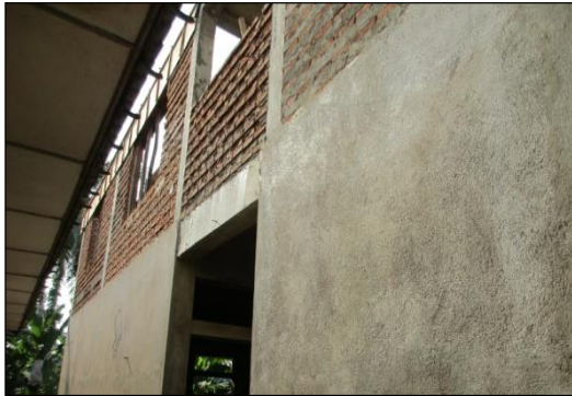
Plastering the walls with cement mortar
