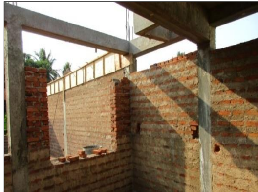
Formwork for beams
