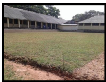
Project: Building a playground in Prince of Wails’ College,
