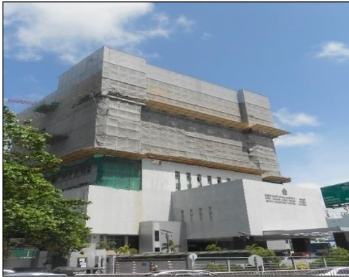
Reinforcement of 16 th floor
