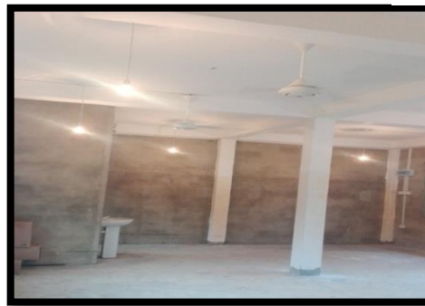
Project: - Completing Praja Shala Building- Kahatapitiya, Seethawaka
