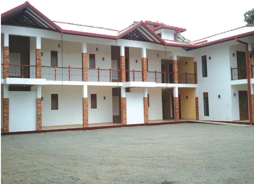
KATARAGAMA NEW REST OPENING
