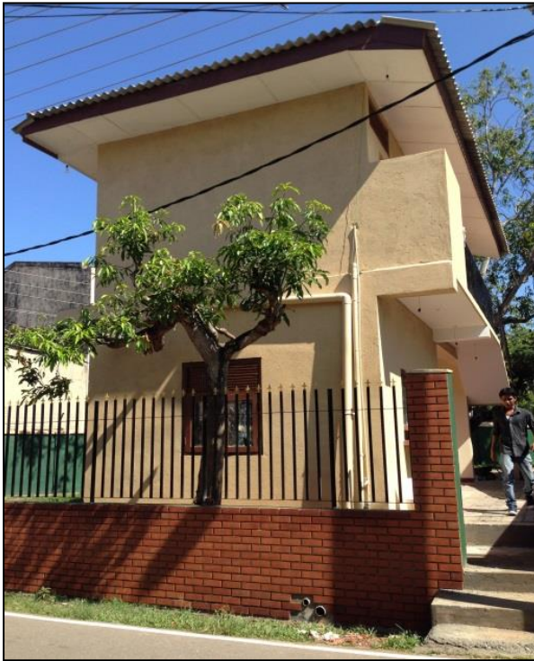
Two Storied Security Building & Hardware Lab at ATI - Dehiwala
