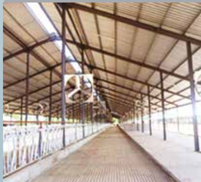
Construction of New Cattle Sheds
