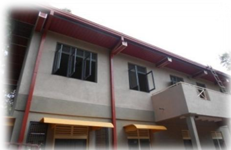
Vidatha Building at Nallur
