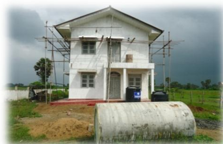
Vidatha Building at Musali
