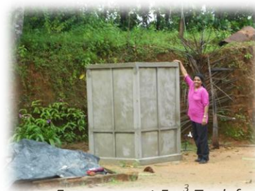
Ferro-cement 5m 3 Tank for Rainwater Harvesting in Kuttivila
