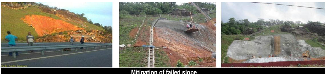
Mitigation of failed slope
