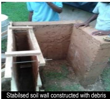
Stabilised soil wall constructed with debris
