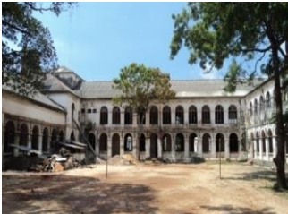
Restoration in progress
