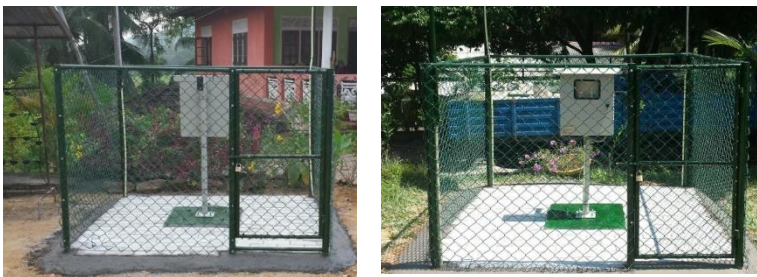
Installation of automated rain gauges in progress in Kithulgoda and Palindanuwara
