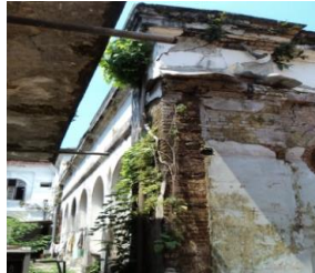
Extent of damage
