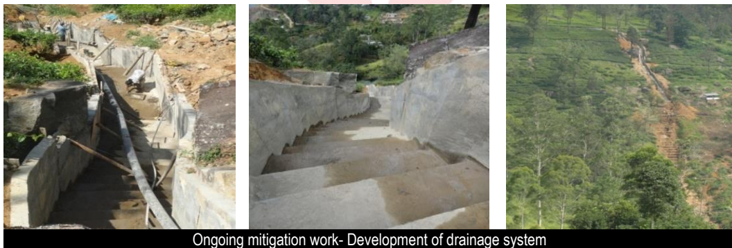
Ongoing mitigation work- Development of drainage system
