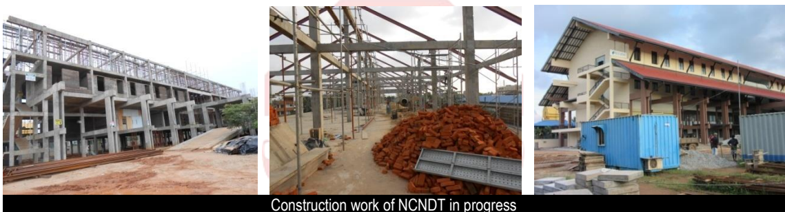
Construction work of NCNDT in progress
