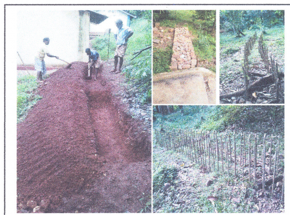
After the Construction of Soil Conservation Demonstration
