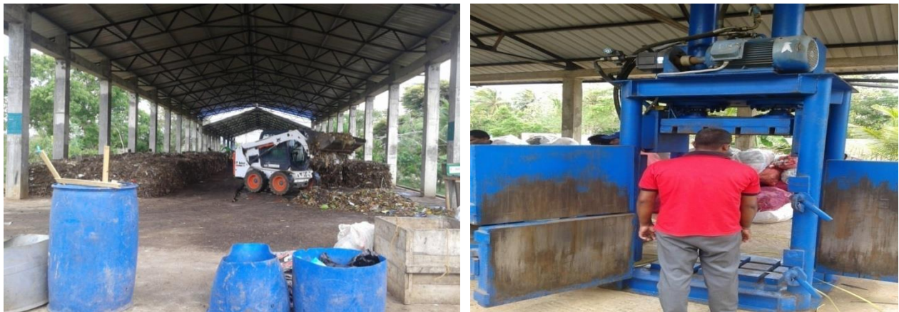
Garbage Disposal Centers – Galgamuwa and Wariyapola
